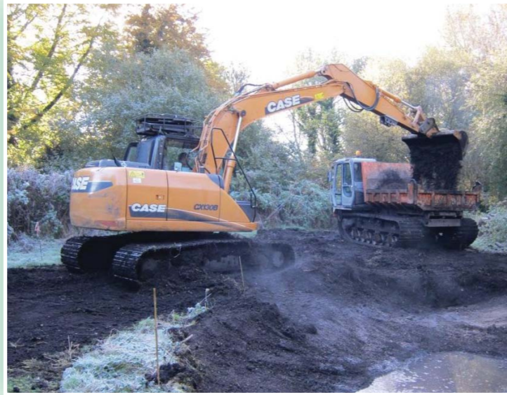
Digging a new pond at Cassiobury Park Nature Reserve © Tim Hill
